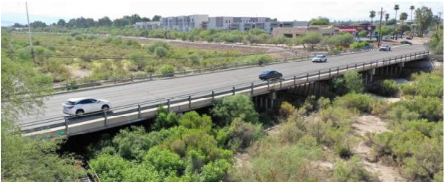
First Avenue Bridge over Rillito Creek
